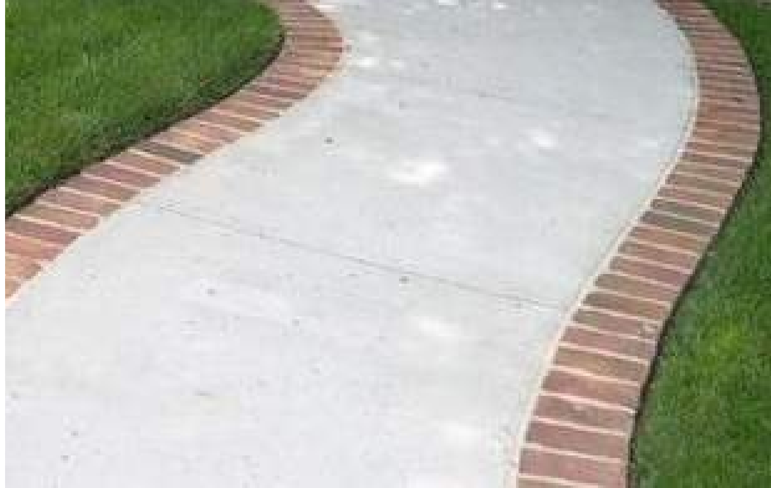
CONCRETE PAVING WITH BRICK PAVER BANDING
