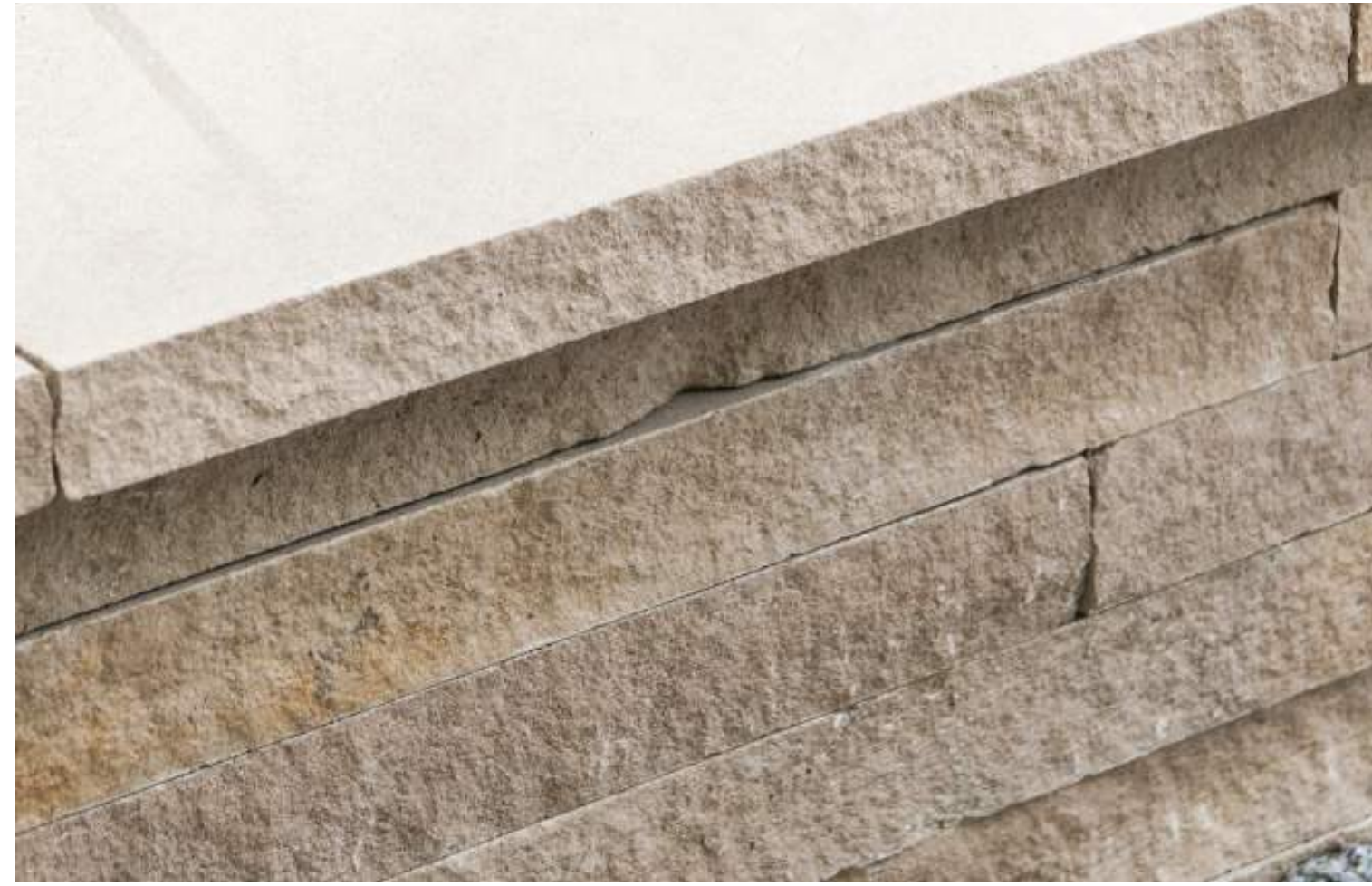
SMOOTH FINISH LIMESTONE SEAT WALL
